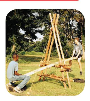
Since the roller spar will eventually be rotating between the A-frames, the actual distance the A-frames are apart is determined by the diameter of the roller spar. Four Scouts should hold the A-frames upright and steady.
